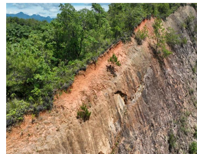
K36+115~K36+290 段路基左侧上边坡滑塌
