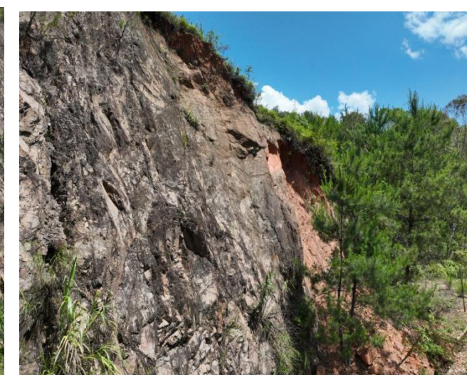
K36+115~K36+290 段路基左侧上边坡滑塌
