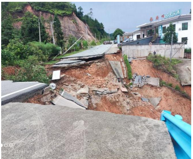
K32+220~K32+320 段路堤垮塌，护栏等防护设施损毁、浆砌拱涵崩塌
